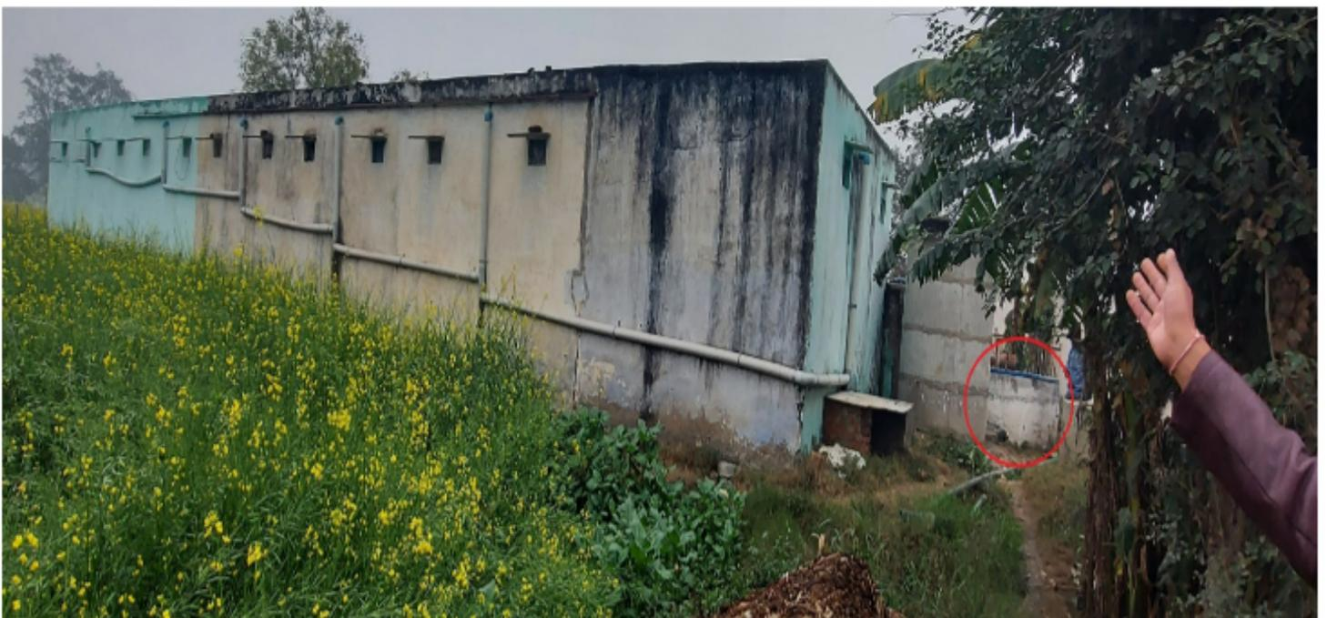
*Collecting water from different roofs for diverting to dry-well (shown in red circle)*
